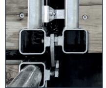
To reduce the space between the docks, you can screw a 2" x 4" board on one side.
